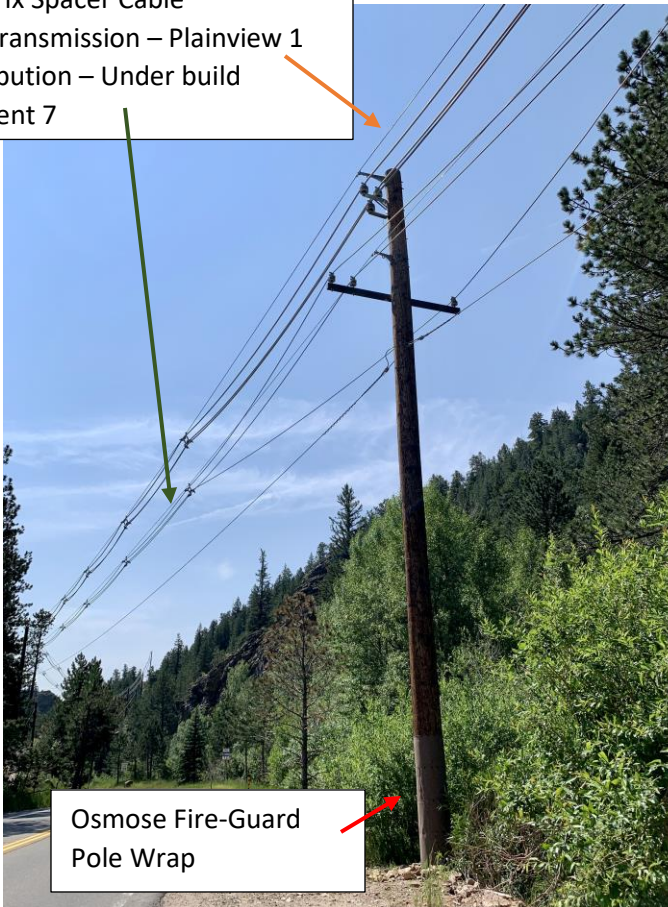
Three-Phase Covered Conductor Blue Mountain 2
