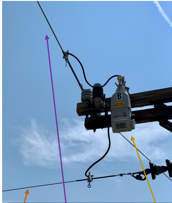
New Covered Conductor and Previous style Copperweld New 'smart' Recloser for isolating the Line
